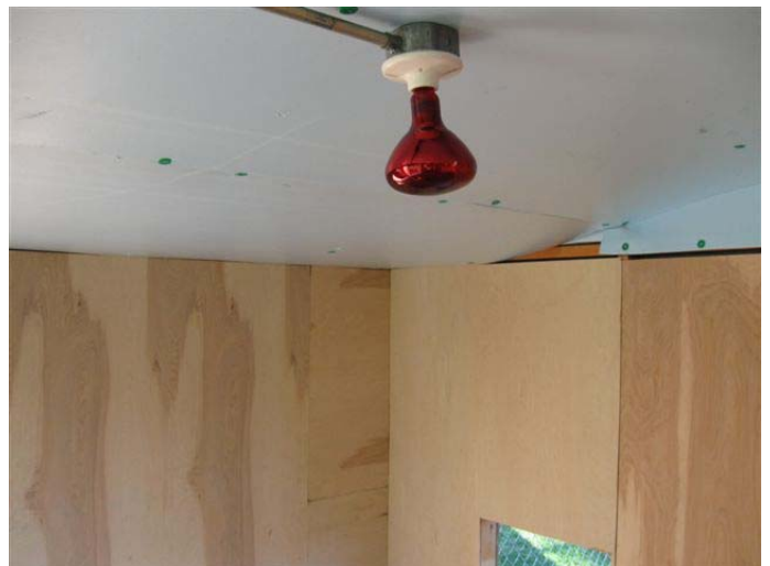
Meg's Place heating element
