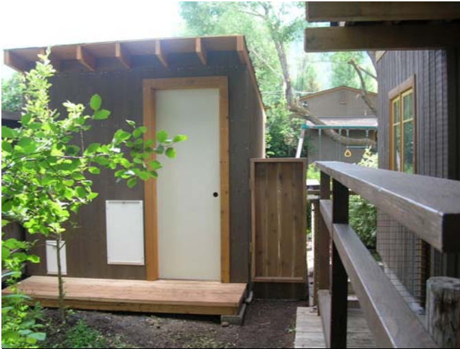
Community Safety Network
