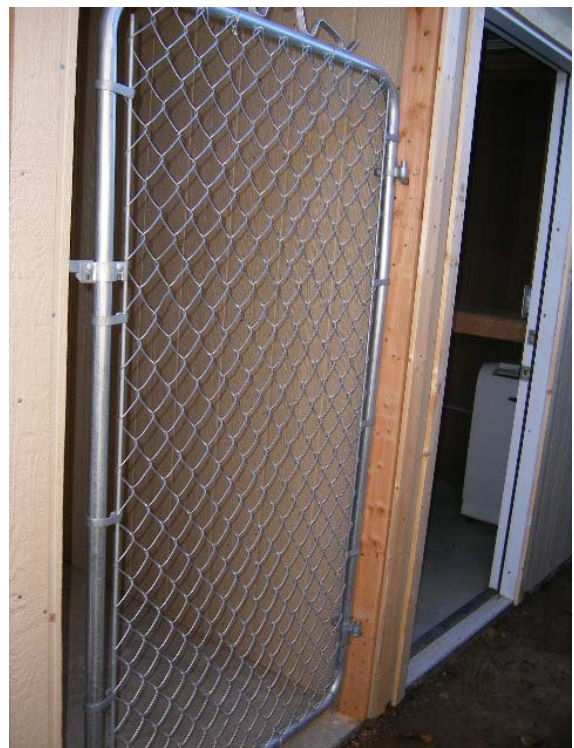
Mt. Graham Safe House
