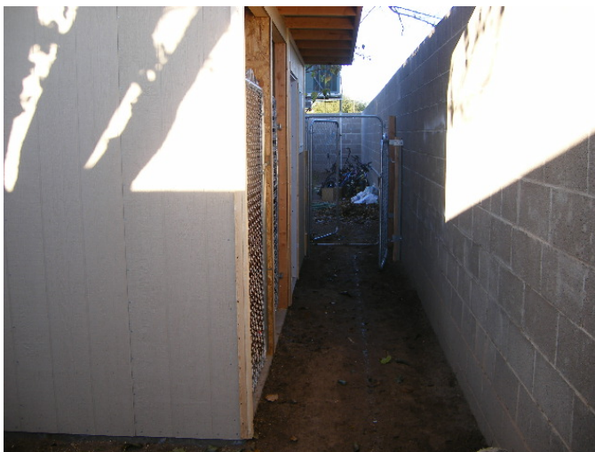
Mt. Graham Safe House
